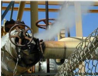
Steam is used in many ways and at various pressures. Sometimes equipment will develop a steam leak. The pressure and temperature of this steam can cause serious burns. Steam leaks at very high pressures can be *invisible and dangerous*.
